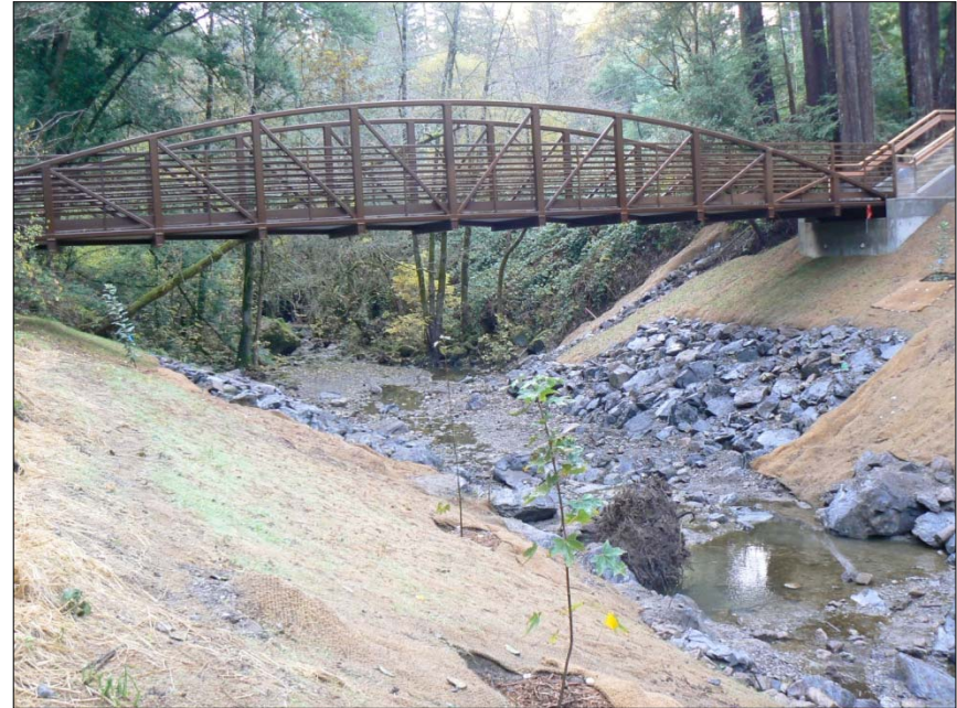
The New Camp Meeker Bridge Photo taken December 1, 2009
